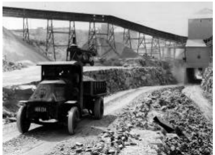
Jamesville Quarry when it was providing limestone for the production of soda ash, 1921.
