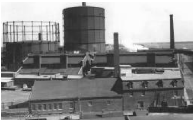
The Consumers' Gas Company water gas purifying buildings (1926) in front of two large gas holders. The short rectangular ventilation shafts identify the building. Source: City of Toronto, Consumers' Gas photographic collection, SC 34 - #340.
