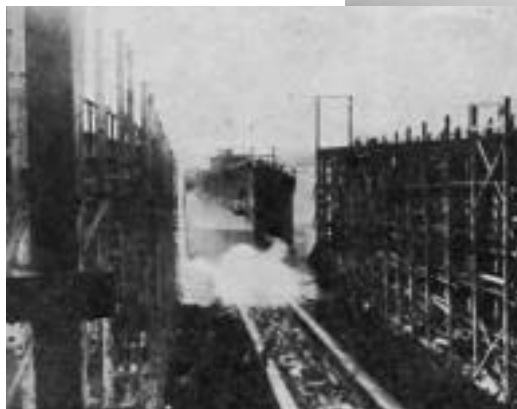
Merchant Shipbuilding launches a “fabricated” freighter. Source: Emergency Fleet News , Sept. 19, 1918.
