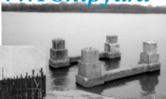
Concrete pedestals are all that remain of a Merchant Shipbuilding shipway in Bristol, PA.
