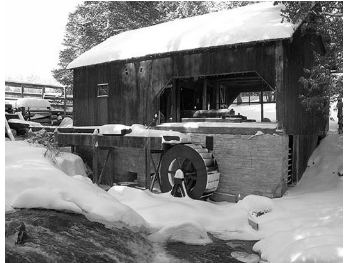
O'Hara Mill, Canada's only known working upright-frame sawmill, has been restored to operating condition.
