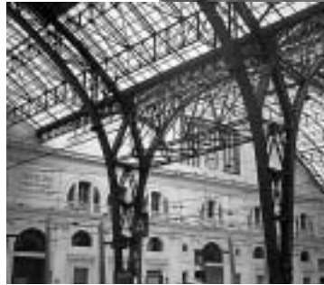
Barcelona Train Shed.
