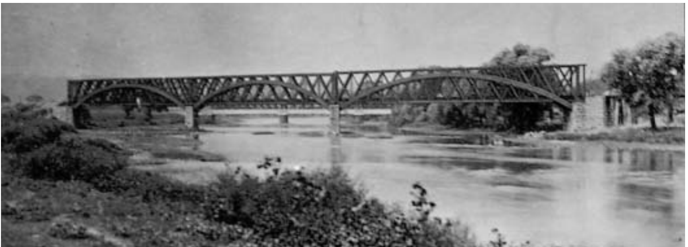
The third Stonerstown bridge, built on shorter piers after the 1874 realignment of the railroad. A series of Howe through trusses.
