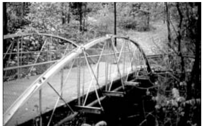
King bowstring truss bridge, Newfield, NY, photo from ca. 1995.
