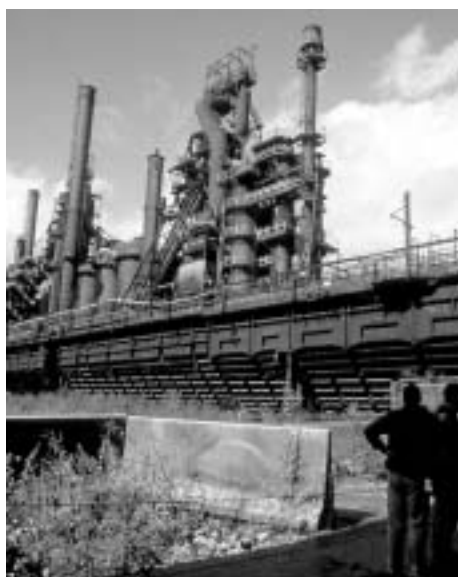
The blast furnaces at Bethlehem Steel. The wide-gauge "Hoover-Mason Line" material-supply railway is in the middle ground.
