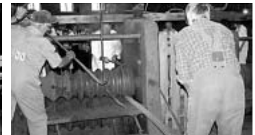
Working the Lancashire forge at Karmansbo: The heated iron is lifted from the hearth onto a small cart (left), transferred to the “mumblingshammer” (middle), then to the rolling mill (right).
