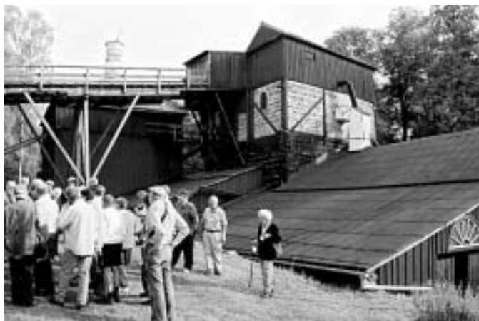
The blast furnace at Engelsbergbruk, built in 1779 and rebuilt in 1878, is one of the few earth-and-timber furnaces preserved in Sweden.
