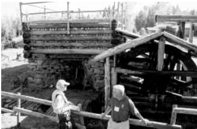
At Nya Lapphyttan, in the mining district of Norberg, a 12th-century blast furnace complex has been recreated based on archeological evidence recovered nearby.
