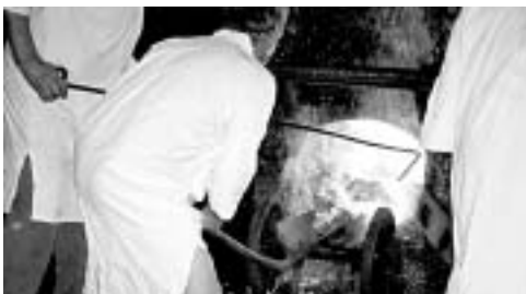
Working the Lancashire forge at Karmansbo: The heated iron is lifted from the hearth onto a small cart (left), transferred to the “mumblingshammer” (middle), then to the rolling mill (right).
