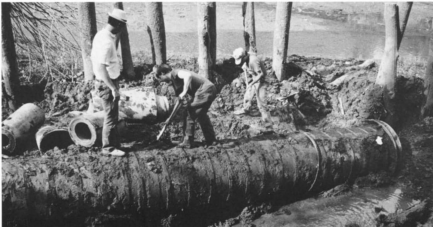
Valentine museum crew (L-R: Lyle Browning, Gregg Kimble, and Greg Galer) removes muck from around the larger of two 1852-53 archimedes screw pumps found in a drained section of the James River & Kanawha Canal, Richmond, Va. Later, the wood-stave pump was lifted out by a Chinook helicopter provided by the U.S. Army Corps of Engineers, whose personnel also had helped dig out the rare 38-ft. artifact. *Photo courtesy of Kathy Franz, Valentine Museum.*
