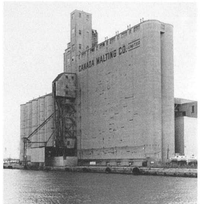
Above: Threatened Canada Malting Co. elevator (1928) in Toronto. Greg Tjepkema photo for Harbourfront Magazine.
