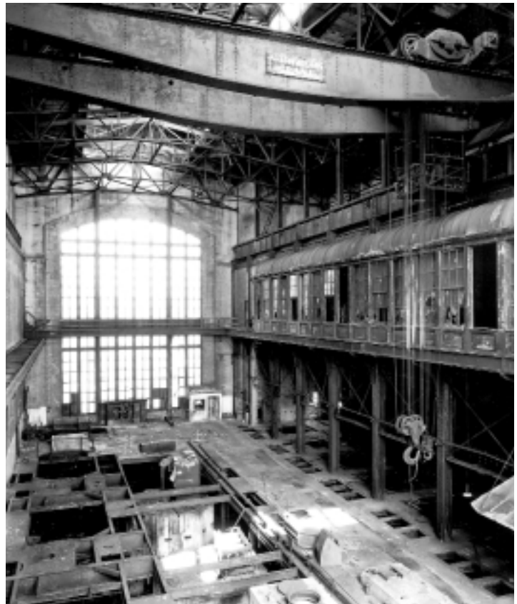
H&M Powerhouse interior view with cranes overhead.
