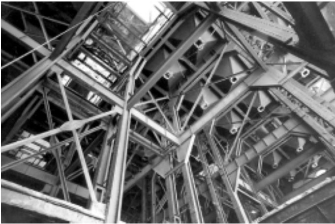
H&M Powerhouse interior steel framework.
